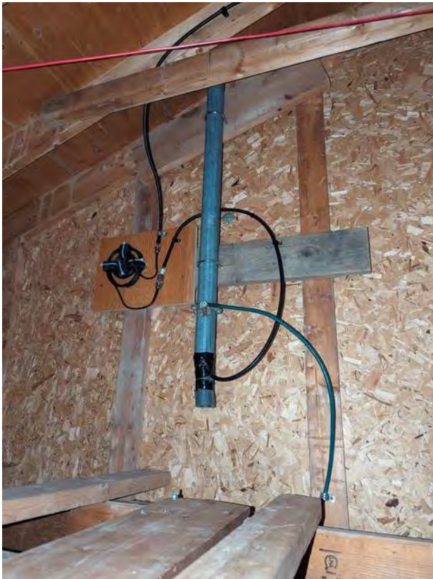
Choke is seen in the inside attic picture. Picture of the back of the house from the road shows the stack at the peak on the left. EFHW attachment stack is just visible at the left roof peak
